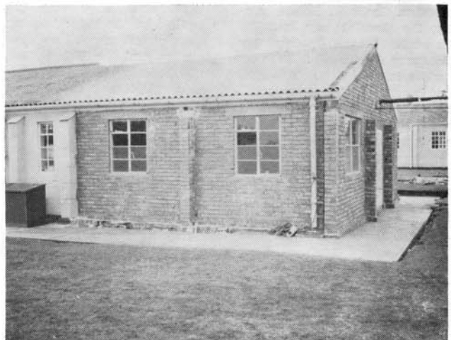
Progress on the extension to the dental building is shown above. Hopefully, it should be completed around the first part of April.
